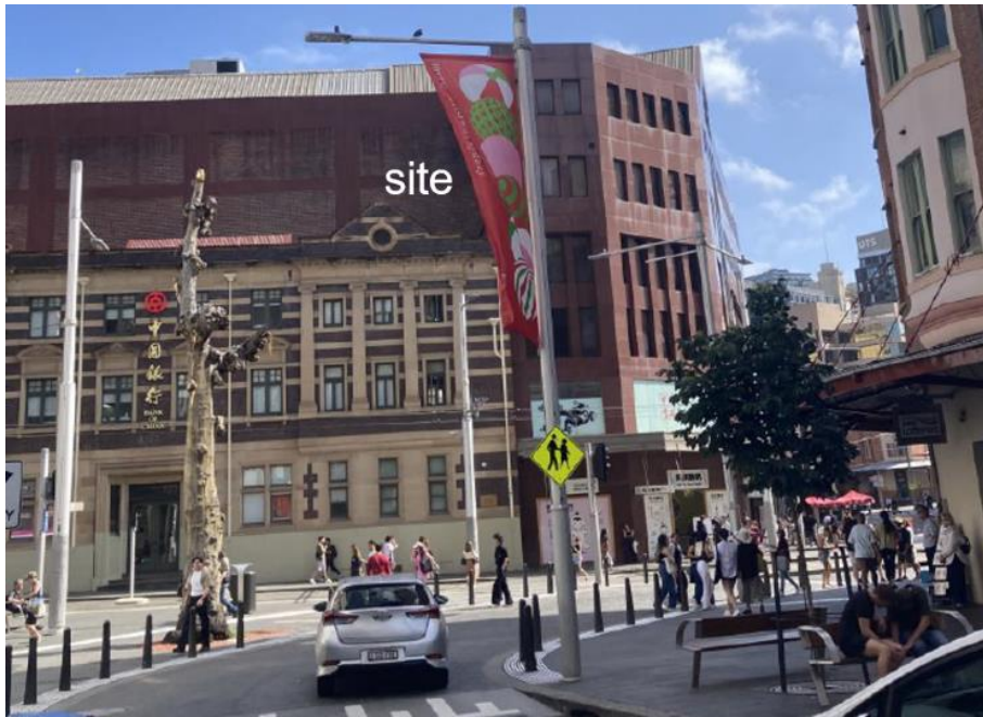
Figure 6: Site viewed from Sussex Street, generally looking south. The neighbouring Bank of China Building is in the foreground.
