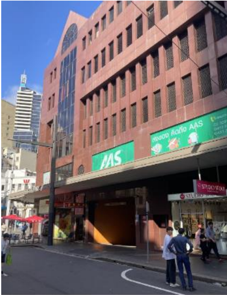
Figure 4: Site viewed from Thomas Street, looking north-east
