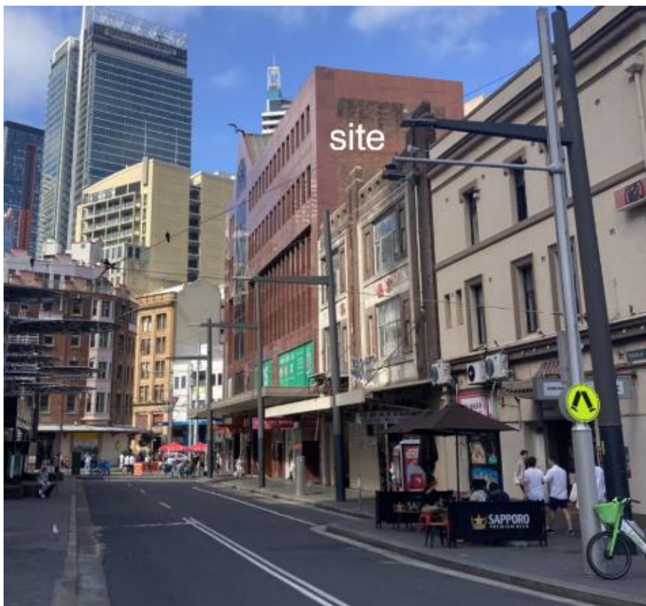
Figure 7: Site viewed from Thomas Street, generally looking north
